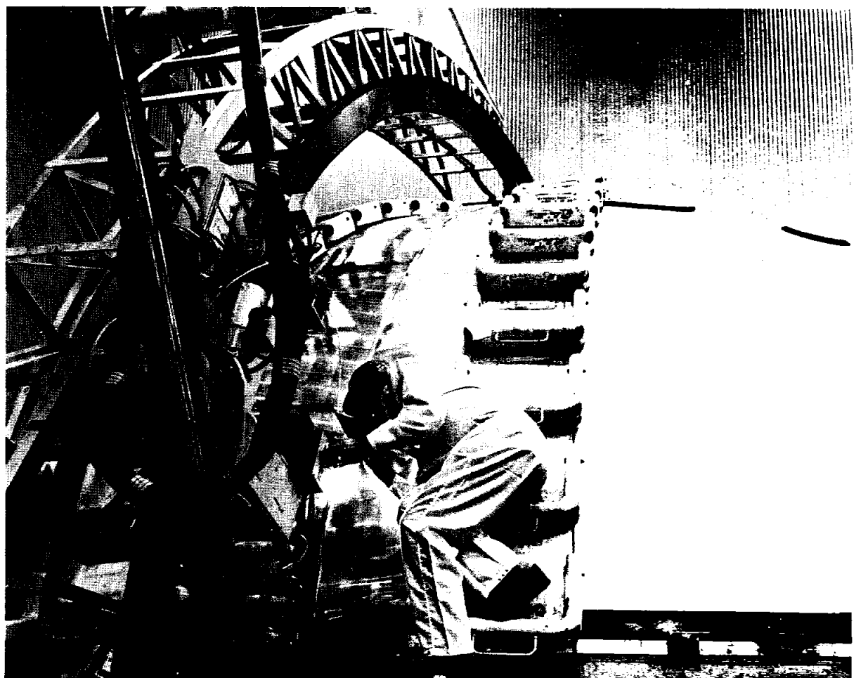
BULKHEAD WELD —The progress of an automatic TIG (tungsten inert gas) weld machine, below, is checked as it welds pie-shaped sections of aluminum together to form the bulkhead, or tank end for one of the fuel tanks for the S-IC.
