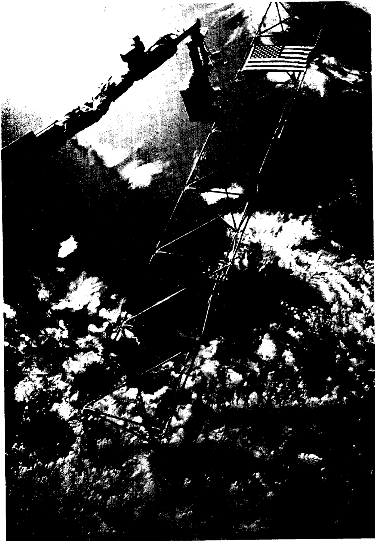
STS 61-B's two spacewalks left little doubt last week that astronauts can effectively and efficiently build large space structures. Out on the robot arm of Atlantis , Woody Spring manipulates the ACCESS truss during the second EVA.
