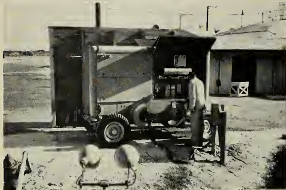
Snark Missile is powered by this Caterpillar Electric Set, photographed at Cape Conover, Florida. Full designation: Caterpillar 60 KW 400-cycle 120-208 Voltage Low Silhouette Portable Ground Support Unit with Precision Control Regulation.
