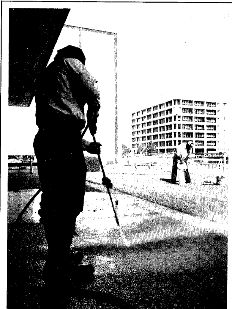
JSC Photo by Bob Walck SPRAY AND WASH —Johnson Controls workers Oscar Aldrete, left and Juan Leon pressure wash the sidewalk outside Bldg. 16. The on-going maintenance program by Center Operations Special Purpose Maintenance and Services Office is designed to wash out the mildew and dirt that build up between the gravel in the sidewalk and on the buildings' walls.
