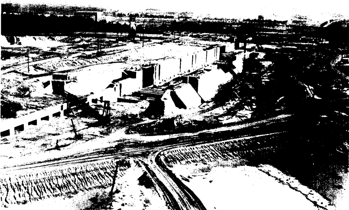
NAVIGATION LOCK —The quarter of a mile long navigation lock with its upstream and downstream guard walls, is shown under construction. The lock will lift the barges with the saturn rockets some 23 feet to the canals that service the test stands. The lock length from gate to gate is 670-feet.
