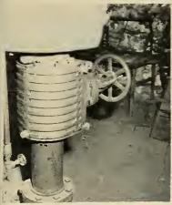
The device is made of two sheets of metal, with the outside sheet embosed to create flow channels. The inside sheet, which is flat, provides greater heat-transmitting contact. The two sheets are welded together and curved to fit the valve.
