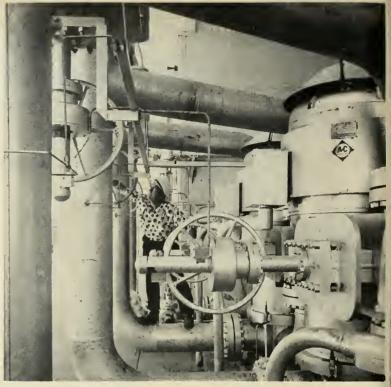
Pipe lines from three multi-stage centrifugal pumps on Rocketdyne's test unit. Harold Hupp sets one of the valves on the equipment, the largest of its kind in the free world.
