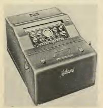
the company, a division of Hamilton Watch Co. The unit, named the S-25C, is a multi-element, all-purpose oscillograph designed for unlimited application, convenience of operation and high-quality recording. The device is cartridge-loaded and uses 12" wide recording paper capable of recording 18 or 48 channels. Circle No. 206 on Subscriber Service Cord.
