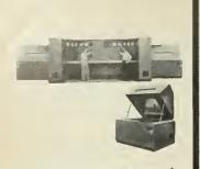
ENVIRONMENTAL CONTROL PANEL AND TWO COLD BOXES USED TO ATTAIN TEMPERATURES FROM AMBIENT TO -65°F IN MISSILE CON-TROL COMPONENTS.
